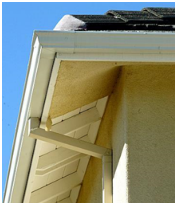
Figure 28. An open eave with no soffit
